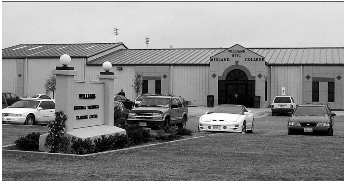
Midland College's Williams Regional Technical Training Center in Fort Stockton
